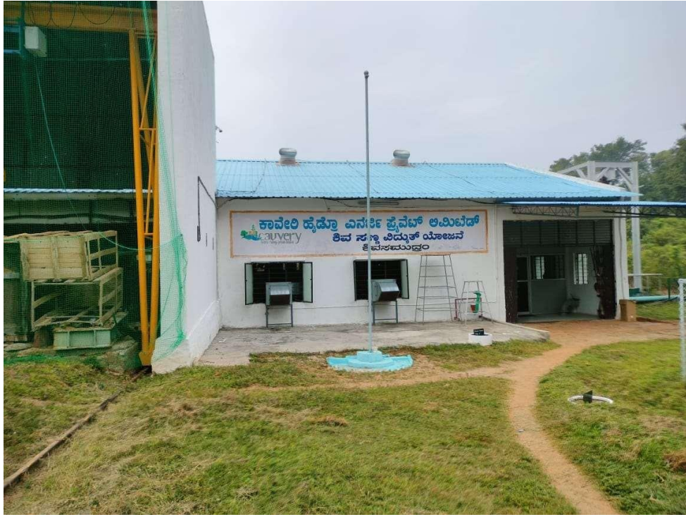
Fig.7 photo at Cauvery hydroelectric power plant
