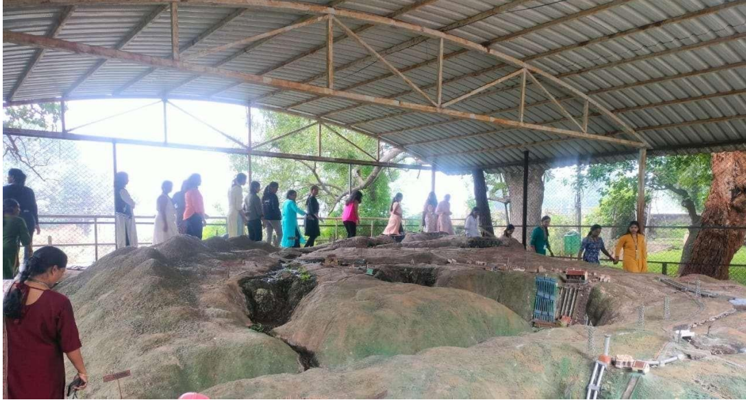
Fig.1 Overview of Hydro power plant
