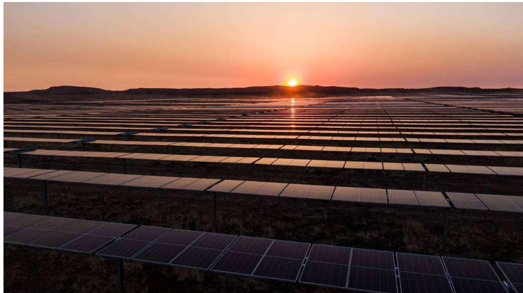
Fig.2 Overview of Solar Power Plant
